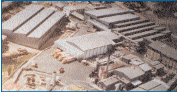
Aerial view of the Bull Brand meat processing facility, one of South Africa's largest and most outstanding beef packers.
